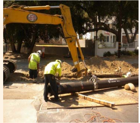
NCWD Construction Crew on Wildwood Canyon, Newhall
